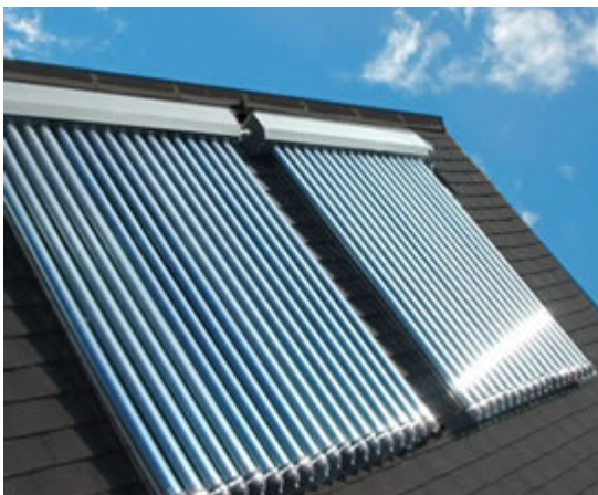
Figure 3 – Example of evacuated tube solar collectors
